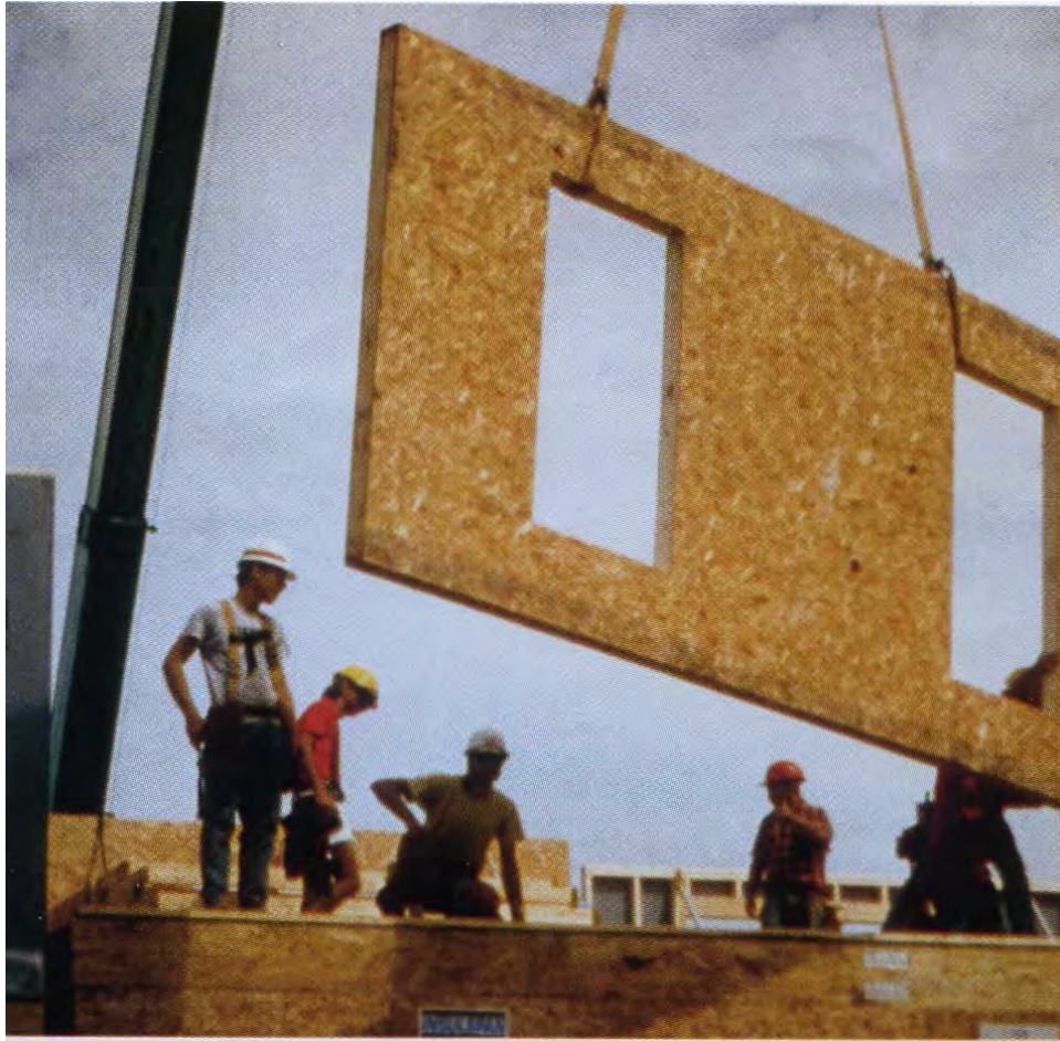
Figure 2.5 Structural Insulated Panel erection. [Morley]
