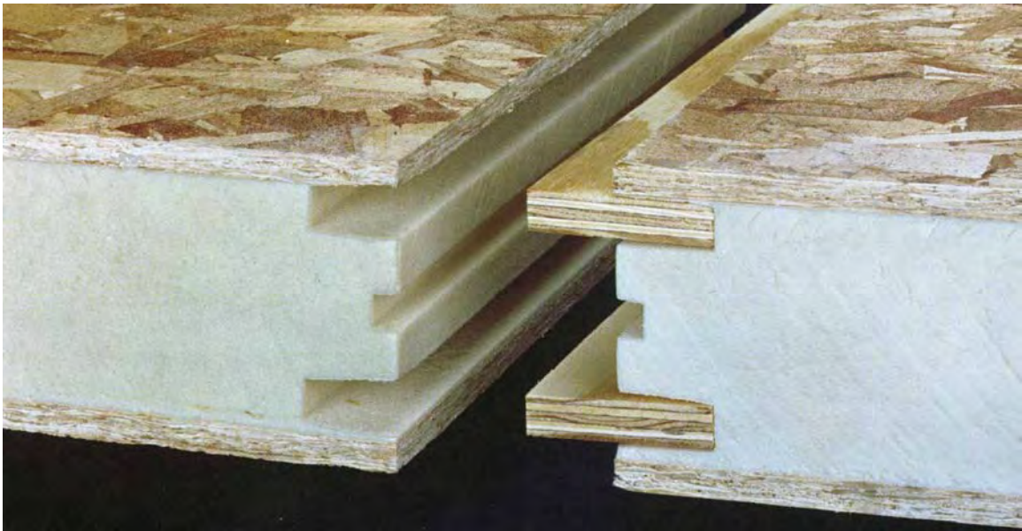
Figure 2.4 Structural Insulated Panel spline joint. [Morley]
