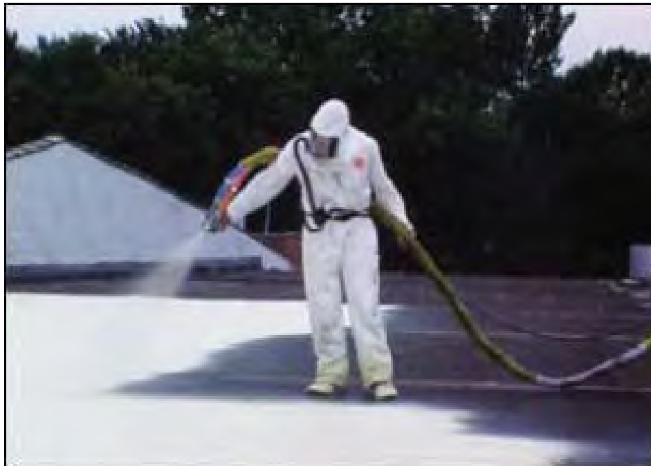
Figure 3.7 Spray application of polyurethane foam. [Moser Roofing]
