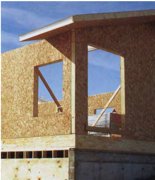
Figure 2.2 Structural Insulated Panel construction. [Morley]
